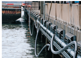
Temporary attachment of the pipe
