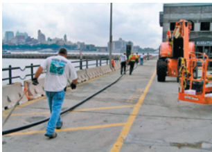
Deployment of 500 ft. of FLEXWELL®-HL pipe
